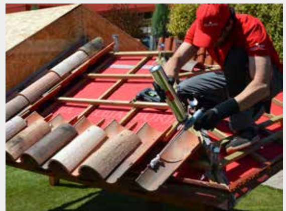
Pre-marked holes to secure the tiles in pan position.
