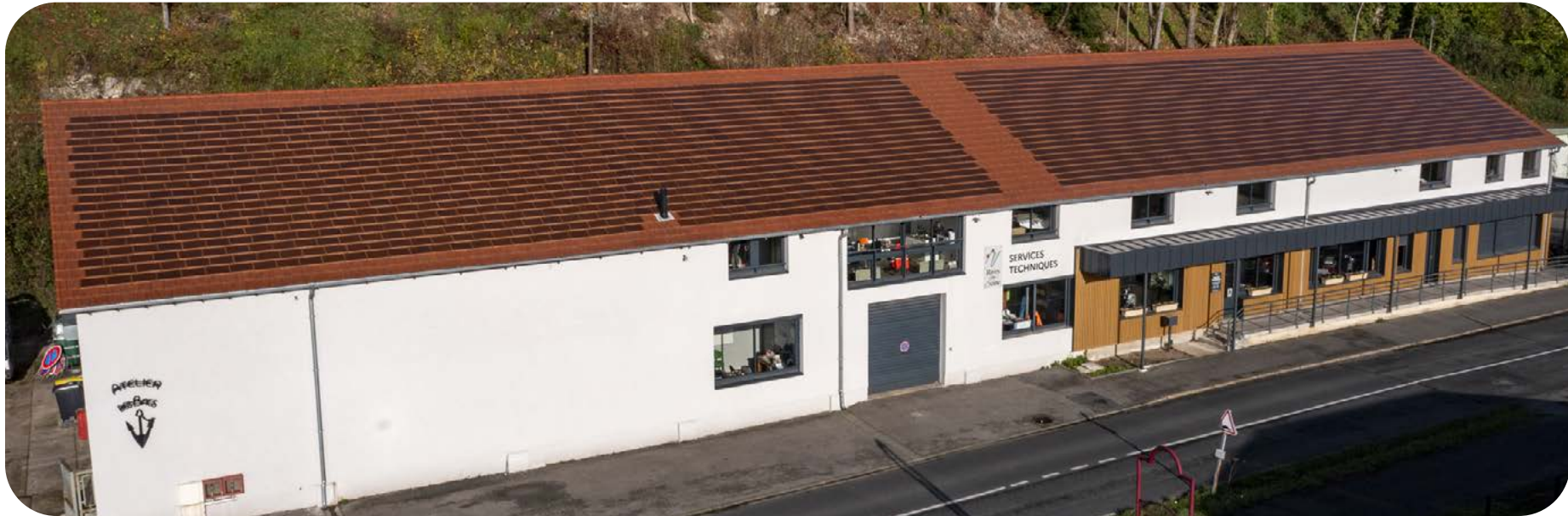
> Overview of the Technical Department Building
